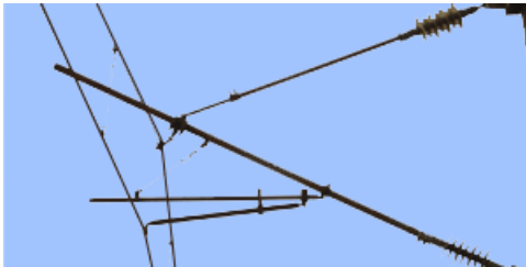
Cantilever Assembly
